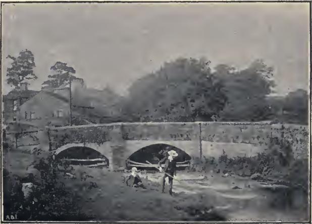
HARDEN BECK BRIDGE.
